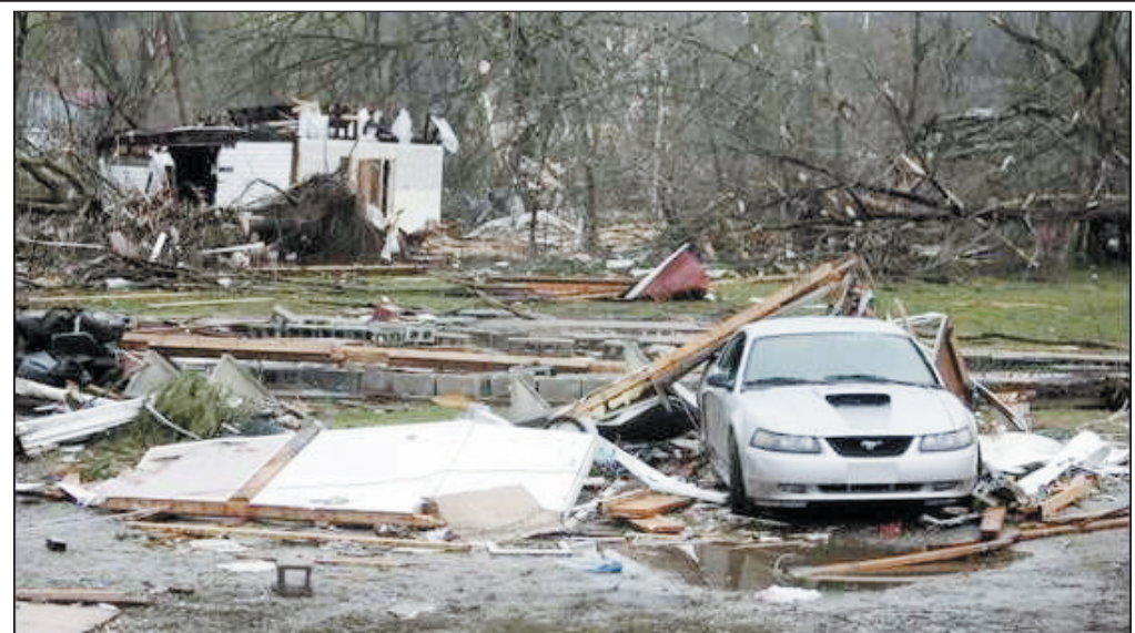
Jeremiah Faulkner's 2003 Mustang was still sitting in the drive-way last Wednesday morning, although all the windows were broke out, but the housing unit where he, his fiancée and two other people lived in two duplexes was completely destroyed by the tornado. Only a few concrete block remained. In the background is another house on the same side of the street that was spared. The people living in the other duplex were killed in the tornado.
