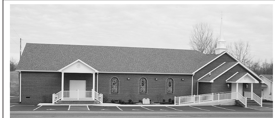
The Hickory Grove Pentecostal Church building has undergone many changes since it was first built in 1954. The church building is located near the intersection of Brindle Ridge and Copper Creek Roads.
