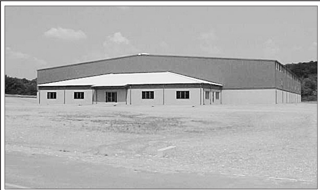
This is an example of how some speculative buildings built to attract businesses to communities look.
