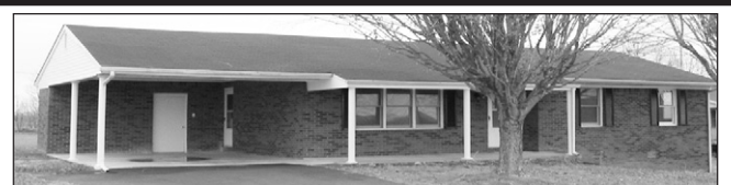
Remodeled 3 bedroom brick, new heat pump, new carpet, new paint. Great view, nice lot. Country location close to Brodhead and Mount Vernon on Union Chapel Rd. $79,900. Extra lot can be purchased with home. Call 606-875-8703 or 606-451-1021
