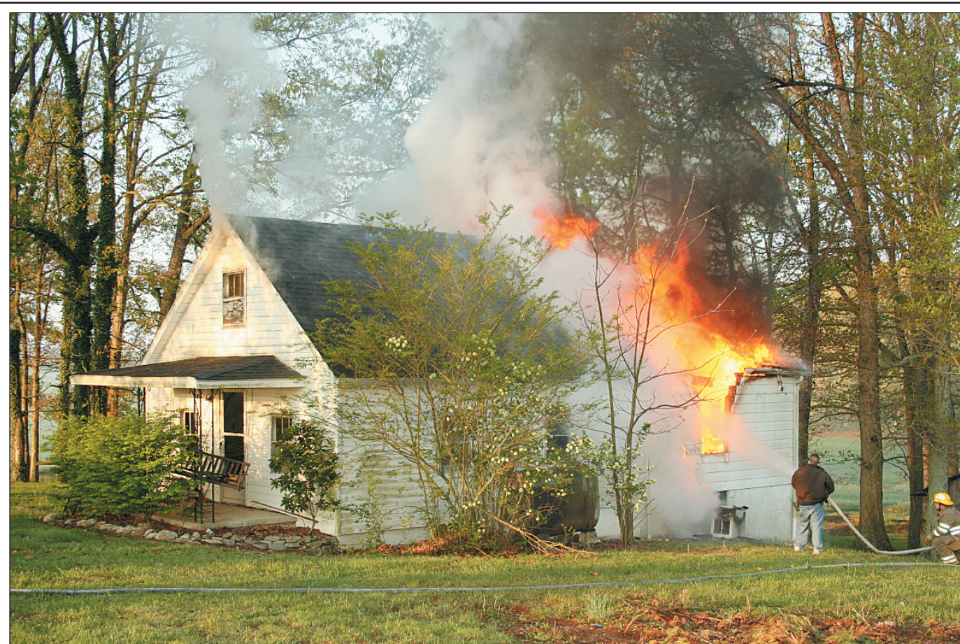
Western Rockcastle Fire Department Asst. Fire Chief Stanley Payne puts water on a fire Wednesday morning, which heavily damaged a house on West Level Green Road between Quail and Bee Lick. Western Fire Chief Johnny Bengé said the house, which is known as the old Foster Brown place and owned by Denver French, was being rented by John Saylor of Copper Creek. The fire started in the back of the house around 7 a.m. Firefighters from Brodhead, Mt. Vernon and Woodstock also responded to the fire call.
