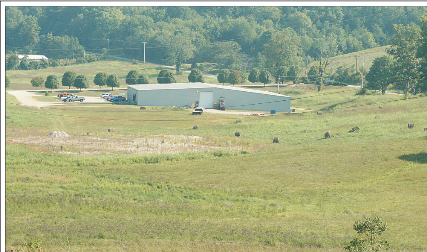
B & H Tool Works, shown in the top photo, will be getting some company when a new 25,000 square foot facility is built in Industrial Park #2 located on White Rock Road, near Mt. Vernon. The facility will house SourceCorp, which has announced an expansion in the county that will create 139 new jobs.
