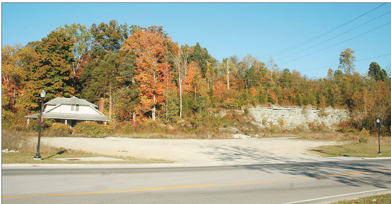
The Mt. Vernon City Council will discuss condemnation efforts on some of the above property located at Renfro Valley. The Rockcastle Tourist Commission says they need the property for right-of-way to 20 acres, which overlooks Renfro Valley, I-75 and Lake Linville, where they want to build a Tourism and Conference Center.
