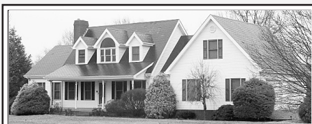
Big & Beautiful! This spacious vinyl sided home at the Rockcastle/Lincoln Co. line has much to offer. Its floor plan could be used as four or five bedrooms. There's also a formal dining room, living room and family room. A two-car garage and additional bay in the basement allow for plenty of space for your vehicle or storage. Call today to view. $190,000. M2423
