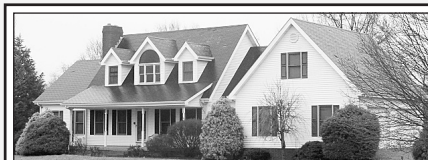
Big & Beautiful! This spacious vinyl sided home at the Rockcastle/Lincoln Co. line has much to offer. Its floor plan could be used as four or five bedrooms. There's also a formal dining room, living room and family room. A two-car garage and additional bay in the basement allow for plenty of space for your vehicle or storage. Call today to view. $190,000. M2423
