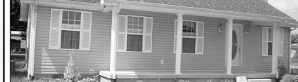
Just Waiting For You! This home consists of 3 bedrooms, 2 baths, kitchen and living room along with a 2-car attached garage. Other amenities include central heat/air, laminate flooring, city water and city sewer. This home sits on a corner lot across from Brodhead Elementary. M2473
