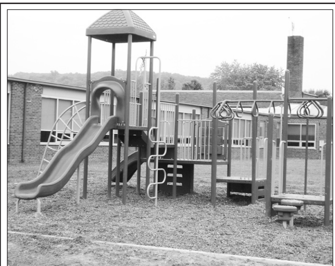
Phase I of Roundstone Elementary School's playground was completed this year.
