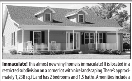
Immaculate! This almost new vinyl home is immaculate! It is located in a restricted subdivision on a corner lot with nice landscaping. There's approximately 1,238 sq. ft. and has 2 bedrooms and 1.5 baths. Amenities include a gas fireplace, 1-car garage, an abundance of cabinet space and a screened-in back porch. $119,000. M2475
