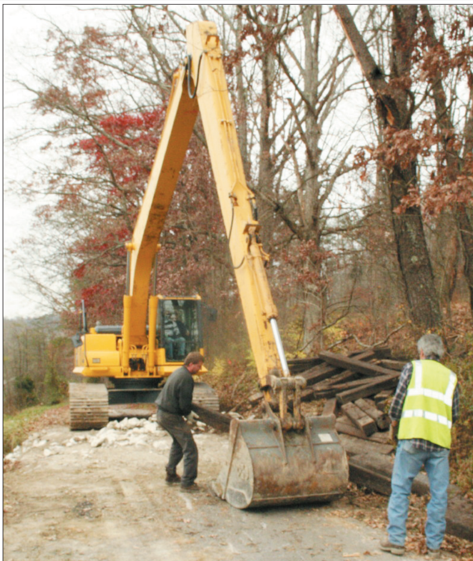
Rockcastle County Road Department employees worked three days last week to repair Boone Gap Road, after a slide made it unsafe to travel the road. The road is located in the northern end of the county off North Wilderness Road. At right, Road Supervisor Coy Cromer, right, and and Gilbert "Spud" Chestnut nail down cross ties donated by CSX Railroad. The ties were put down to help hold the side of the roadway which had slipped away. Above, road department employees Harry Potter and Billy Mason load cross ties into an excavator being operated by Roy Bullock. Cromer said the repairs to the road cost approximately $4,500, not including the 150 man hours.
