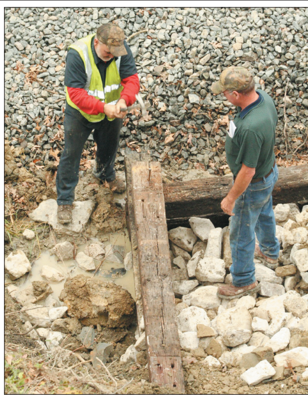
Rockcastle County Road Department employees worked three days last week to repair Boone Gap Road, after a slide made it unsafe to travel the road. The road is located in the northern end of the county off North Wilderness Road. At right, Road Supervisor Coy Cromer, right, and and Gilbert "Spud" Chestnut nail down cross ties donated by CSX Railroad. The ties were put down to help hold the side of the roadway which had slipped away. Above, road department employees Harry Potter and Billy Mason load cross ties into an excavator being operated by Roy Bullock. Cromer said the repairs to the road cost approximately $4,500, not including the 150 man hours.
