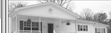
Within city limits! Check out this home with 1,300 sq. ft. +/-, 2 bedrooms, 1 bath, living room, and kitchen. Amenities include stainless steel appliances, maple cabinets, hardwood floors, and city water/sewer. This home is situated on approx. 2 acres and is conveniently located within city limits. Priced at only $89,900. M2526
