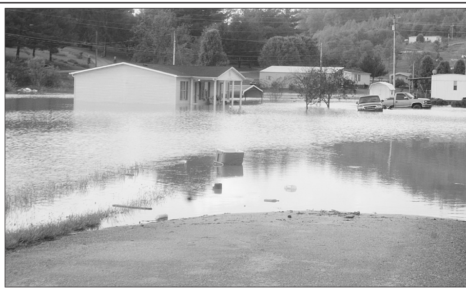
Residents on Freedom School Rd. reported four feet of water in some of their homes after torrential rains fell over the weekend. Many basements in the county were flooded as well as numerous roads being washed out during the rain. County Judge-Executive Buzz Carloftis issued a state of emergency for Rockcastle County.
