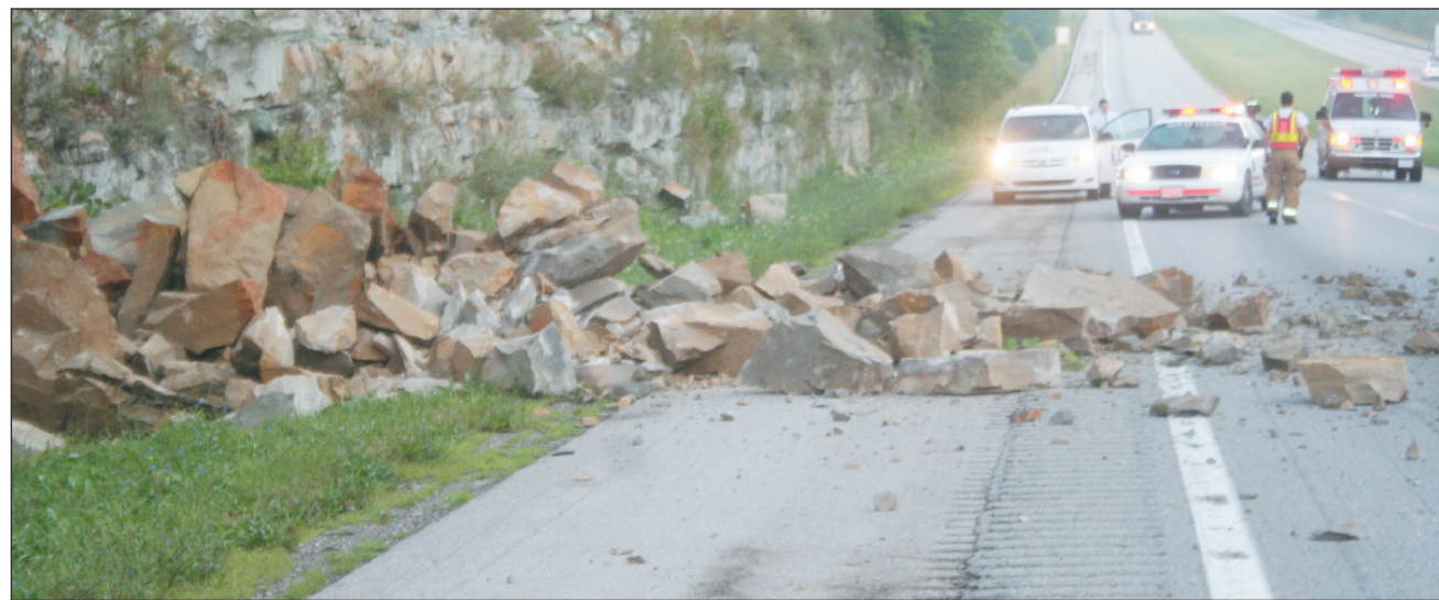
A rockslide in the southbound lanes of I-75 triggered an accident involving five vehicles around 6:00 a.m. last Thursday morning. The most significant accident was of a semi that lost control, crossed the median, flipped and slammed into a rock wall on the northbound side of the interstate. The driver of the semi, from Denton Trucking in McCook, Illinois, escaped serious injury. A load of lumber the semi was hauling was spread across the median and both northbound lanes. Other cars involved in the rockslide reported severe suspension damage and flattened tires. Both southbound and northbound lanes were completely clear by 12:30 Thursday afternoon. Members of the Mt. Vernon Fire Department assisted at the scene.
