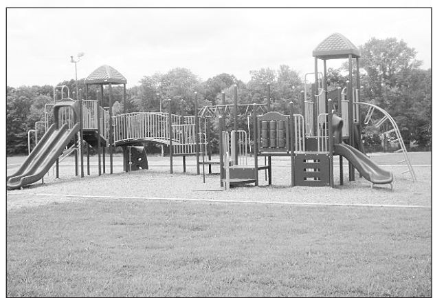
Completed playground for 3rd, 4th, and 5th grade students at Roundstone Elementary.
