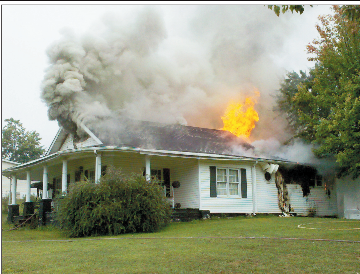
The home of Mark and Linda Callebs on Elsie Lane off of South Wilderness Road was heavily damaged Monday morning by fire that was suspected to have started in the kitchen. Mt. Vernon Fire and Rescue responded to the call as well as the Livingston Volunteer Fire Department. The home suffered major water and smoke damage.
