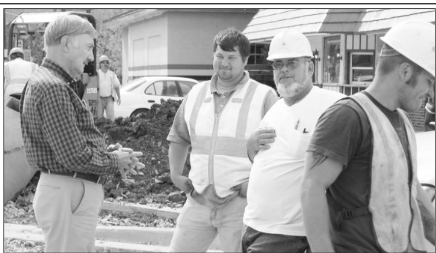
Newcomb Ave./School St. Project is about 75% completed
