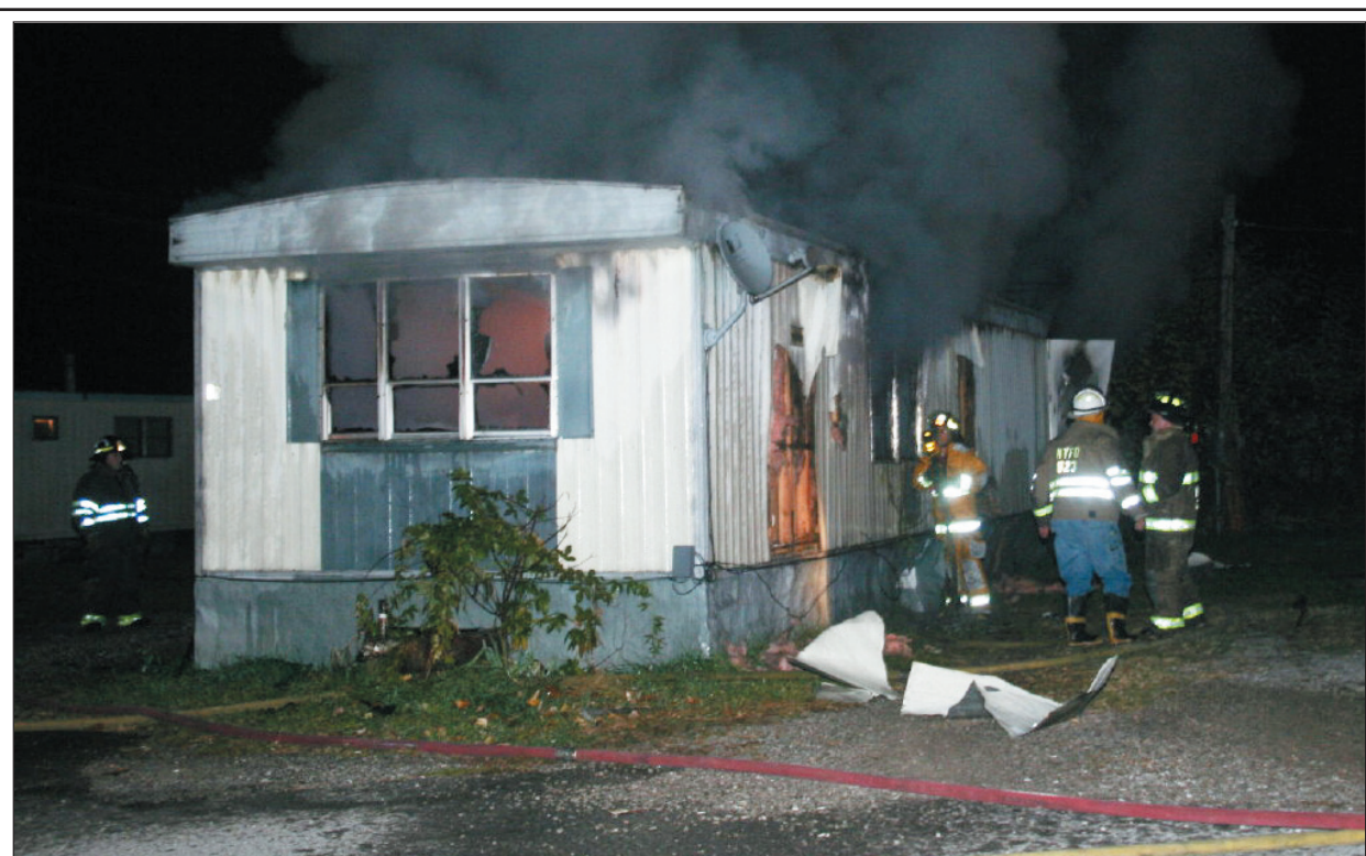
A house trailer belonging to Peggy Bowling in the City Trailer Park in Mt. Vernon was completely destroyed last Wednesday night by fire. The trailer was being rented at the time. The Mt. Vernon Fire Department responded to the fire.
