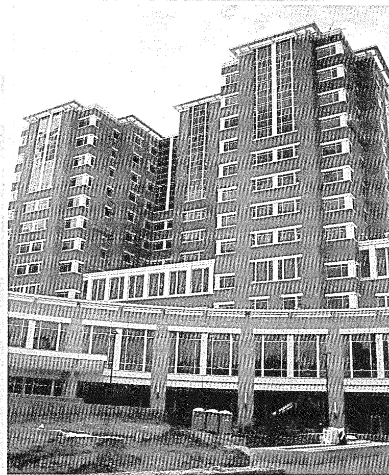
The new Pavilion at the UK Chandler Hospital is on target for a May 2011 opening.
