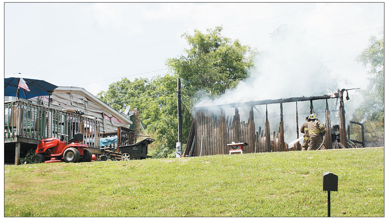
Fire destroyed a large building on the property of Billy Lewis on Carter Ridge Road in Mt. Vernon Monday afternoon. The fire was so hot that it melted the siding from the side of Lewis' home. Noone was injured in the fire. Mt. Vernon Fire and Rescue responded to the scene and put the fire out.
