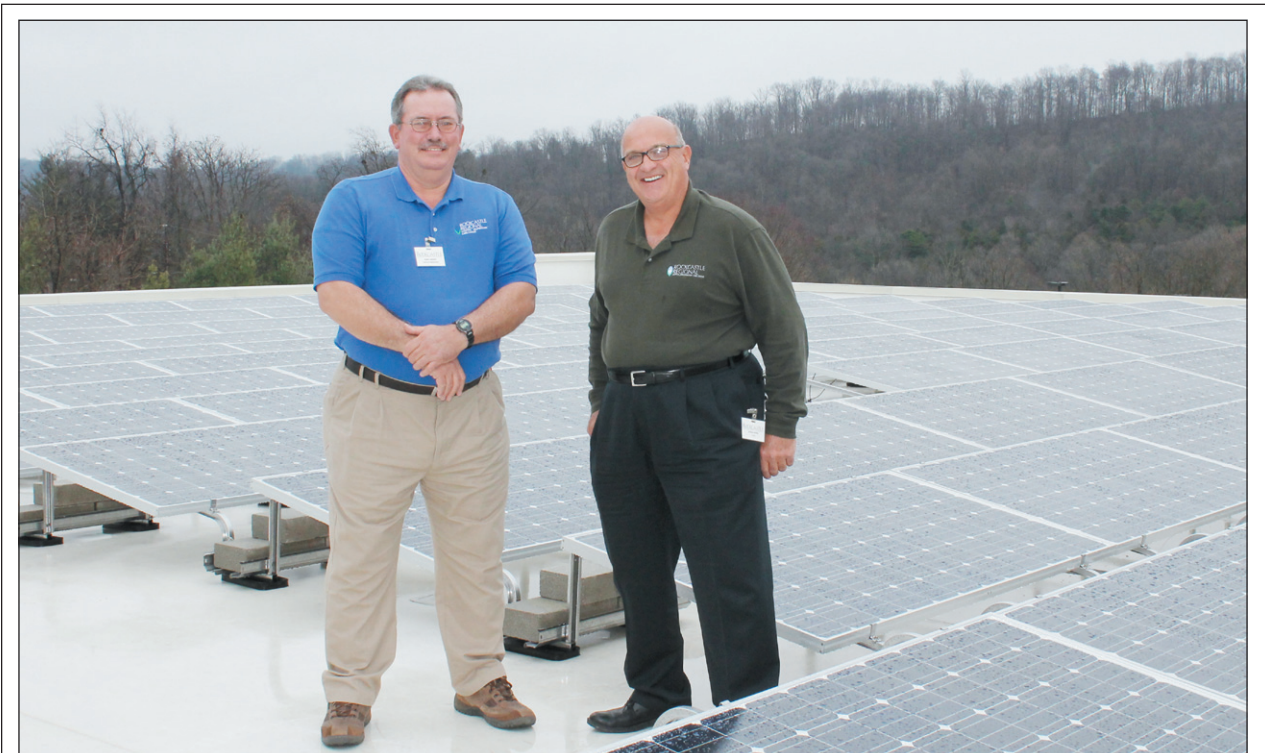
Rockcastle Regional Hospital and Respiratory Care Center went live with solar power on November 30th. Gary Asher, Facilities Manager, left, and Stephen A. Estes, CEO, stand near the new solar array on top of the hospital's Outpatient Services Center.
