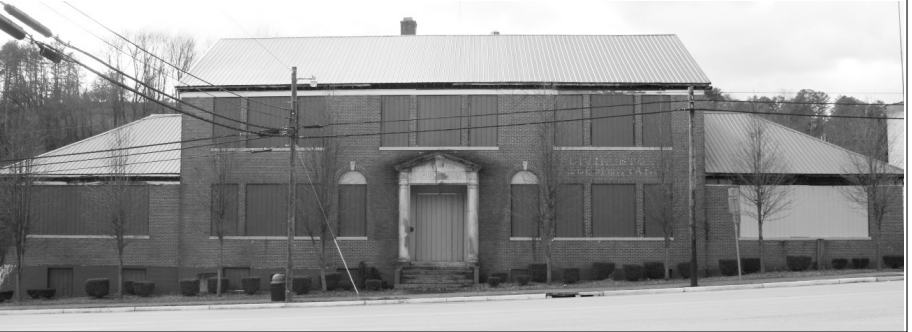
The old Livingston school building where the Livingston Revitalization Committee hopes to remodel some of the rooms to use for offices.
