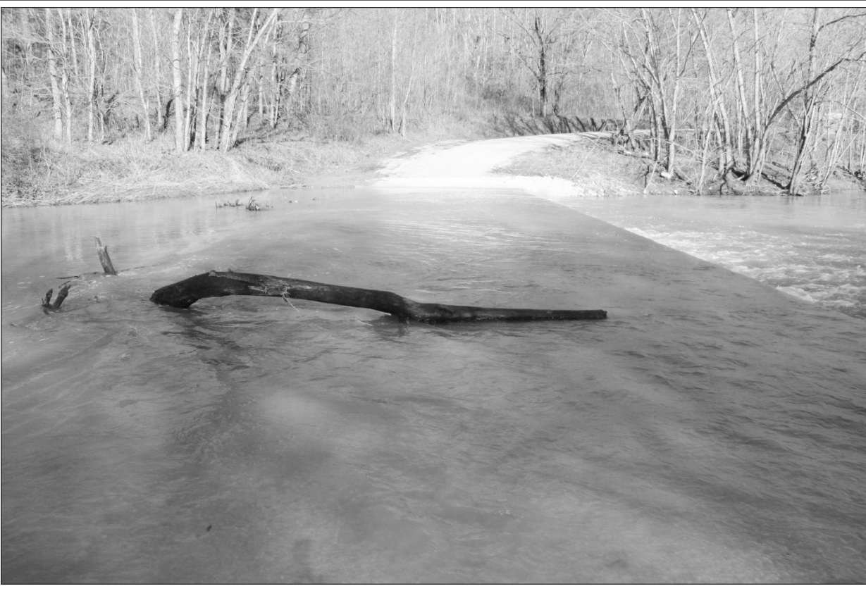
After Friday night's storms, Ten Foot Hole Road in Livingston was unpassable to drivers as water from the Rockcastle River and a tree branch covered the bridge early Saturday morning.
