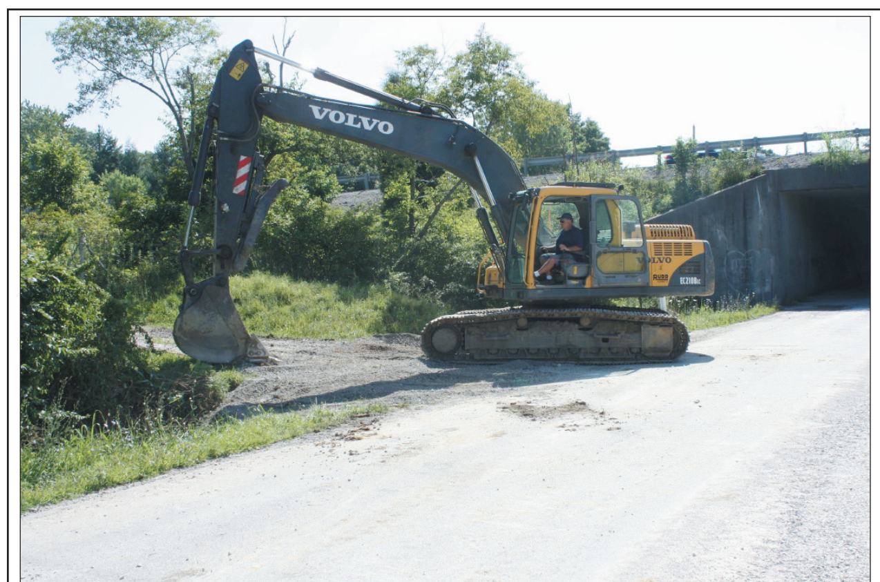
Above, an employee of B&M Construction is shown working on the final one mile segment of Lambert Road. B&M was the successful bidder on the final segment at $48,500. At right shows how much the road was widened during the much-needed project with the area added at the left in the photo. The total three mile project included widening, installing culverts and a new ditch line. Two miles of blacktop for the road has been approved by the fiscal court at a cost of $231,000. County Judge/Executive Buzz Carloftis said he expects the blacktopping to begin within a week after all the "soft spots" in the road are located and repaired. Total cost of the project is expected to be around $600,000.
