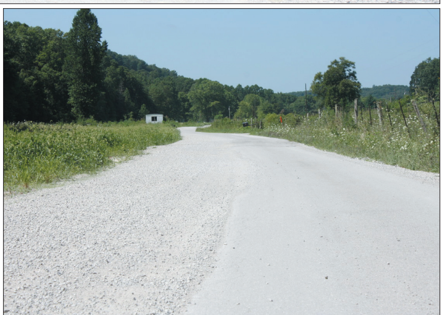
Above, an employee of B&M Construction is shown working on the final one mile segment of Lambert Road. B&M was the successful bidder on the final segment at $48,500. At right shows how much the road was widened during the much-needed project with the area added at the left in the photo. The total three mile project included widening, installing culverts and a new ditch line. Two miles of blacktop for the road has been approved by the fiscal court at a cost of $231,000. County Judge/Executive Buzz Carloftis said he expects the blacktopping to begin within a week after all the "soft spots" in the road are located and repaired. Total cost of the project is expected to be around $600,000.
