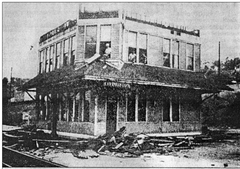
LIVINGSTON DEPOT BEING TORN DOWN --Bill Moore, Bill Smith, Preston Smith in the Windows--
