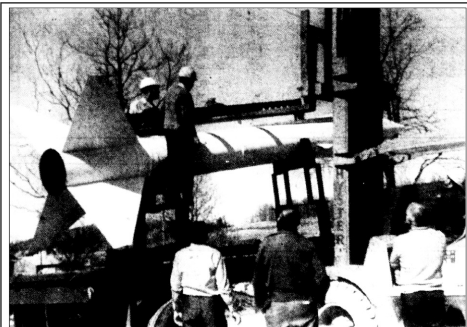
The Clow Corporation of Brodhead donated their time and equipment to unload the rocket at RCHS from the Blue Grass Army Depot. Pictured are Bill Cass and Hershell Woods on the rocket and Charles Lawrence on the forklift.
