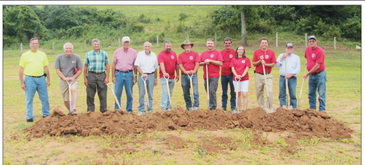
The Climax Volunteer Fire Department had their ground breaking last Saturday for their new fire department building on Hwy 1912 in Climax. The building is scheduled to be completed by November. Shown above from left are: CVFD Fire Chief John Guilfoil, County Judge Executive Buzz Carloftis, Magistrate Gary Burdette, Magistrate Ralph Allen, board member Ken Holt, CVFD Assistant Fire Chief Danny Allen, board member Gerald Chasteen, CVFD Captain Brian Wynn, vice-president Dennis Clark, secretary Denise May, president James Ballinger and board members Virgil Mullins and Steve Hill.
