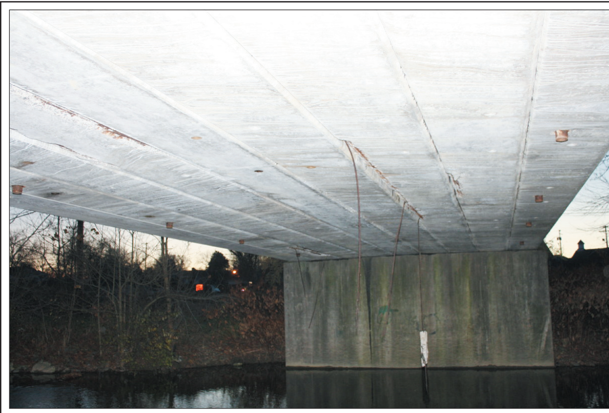
The Dix River Bridge in Brodhead was permanently shutdown last Friday by engineers and bridge inspectors with the Kentucky Transportation Cabinet. Inspectors performed a routine bridge inspection on Thursday and realized the center box beam was deteriorating at a more rapid pace than what they had originally anticipated. Inspectors covered the small hole along the center line with a large metal plate until KTC engineers could inspect the bridge last Friday morning. When KTC engineers arrived, they surveyed the bridge and determined that the center box beam had severely decayed and the bridge posed an immediate threat to drivers. Engineers asserted that if the bridge was left open it could collapse at any given time. Shown above is a picture underneath the bridge that shows exposed rebar drooping from the center of the bridge like tree vines.
