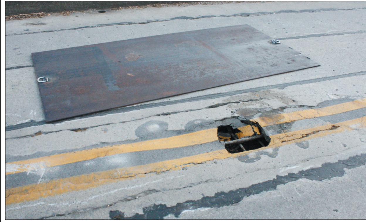
The Dix River Bridge in Brodhead was permanently shutdown last Friday by engineers and bridge inspectors with the Kentucky Transportation Cabinet. Inspectors performed a routine bridge inspection on Thursday and realized the center box beam was deteriorating at a more rapid pace than what they had originally anticipated. Inspectors covered the small hole along the center line with a large metal plate until KTC engineers could inspect the bridge last Friday morning. When KTC engineers arrived, they surveyed the bridge and determined that the center box beam had severely decayed and the bridge posed an immediate threat to drivers. Engineers asserted that if the bridge was left open it could collapse at any given time. Shown above is a picture underneath the bridge that shows exposed rebar drooping from the center of the bridge like tree vines.
