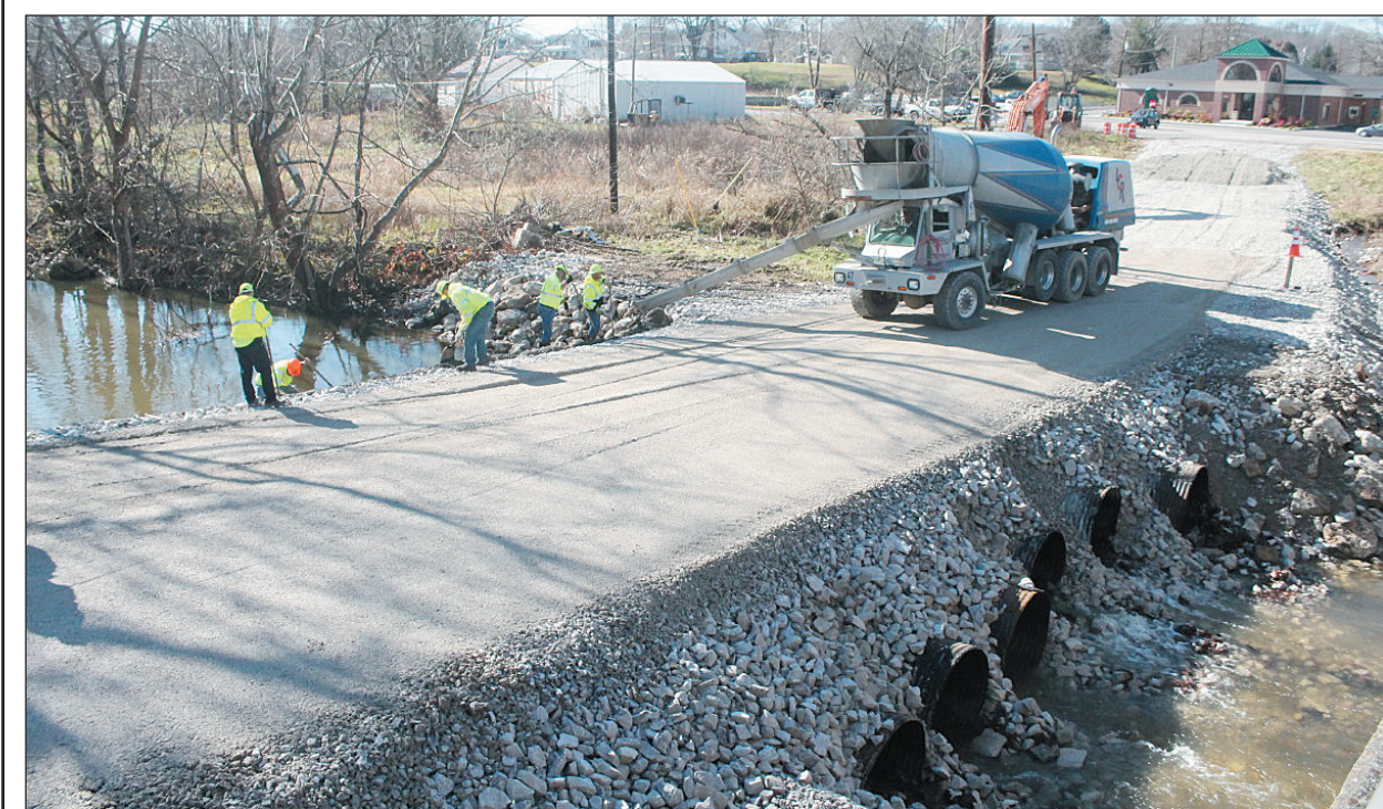
A temporary bridge has been built in Brodhead to eliminate the lengthy detours for motorists caused by the closing of the Dix River Bridge. Kentucky Transportation Cabinet (KYTC) crews started working on the temporary bridge last Thursday and it was completed Monday afternoon. Shown above are KYTC crews pouring concrete on the bridge and shown below is a motorist driving on the bridge after it was opened. The temporary bridge will be in operation until the Dix River Bridge is reconstructed and opened for use. Bids for the reconstruction will be let in January and the project is scheduled for completion in the Spring of 2014.
