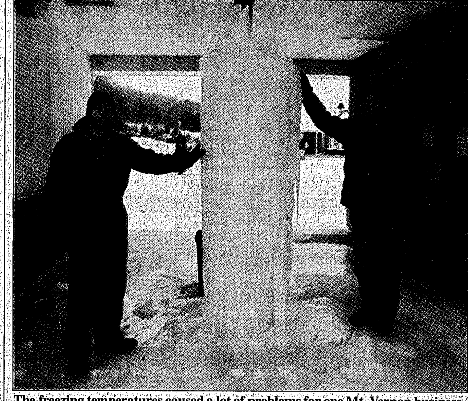
The freezing temperatures caused a lot of problems for one Mt. Vernon business. Businessman Marcus Reppert discovered this large icicle and ice skating rink in one of his car wash bays at his car wash on Hwy 150 in Mt. Vernon. Reppert said a broken valve on top of the spraying wand leaked Tuesday night and Wednesday morning creating the icicle. Reppert is shown with his father Gary Reppert.
