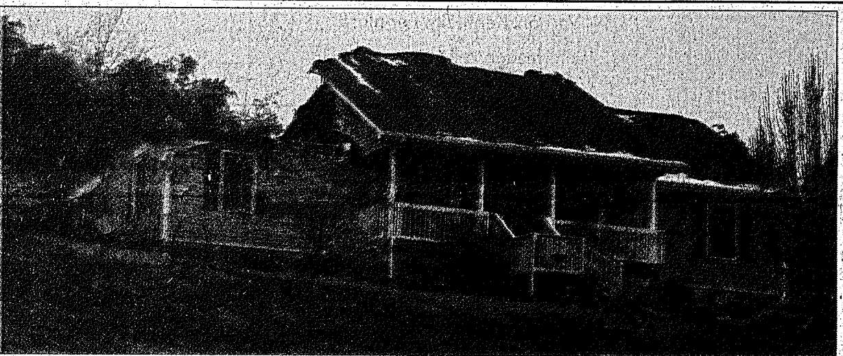
Mt. Vernon Fire Department responded to a house fire Sunday morning on Sawgrass Lane in Mt. Vernon. Authorities say the home belonged to Anthony and Elizabeth Sims. The house was considered a total loss but firefighters were able to salvage a lot of personal belongings from inside the home. The cause of the fire remains unknown and no one was injured in the fire. Mt. vernon Fire Department was assisted by Brodhead Fire Department and Brindle Ridge Fire Department.
