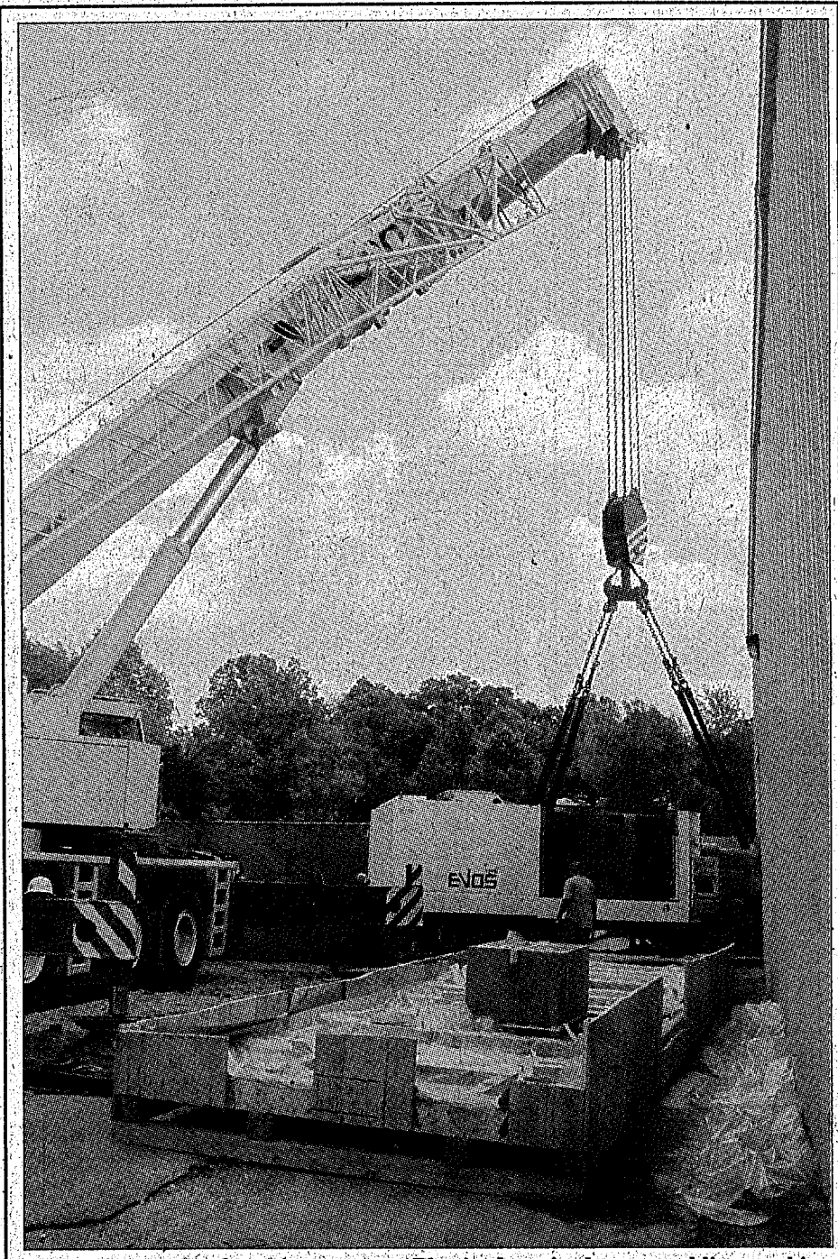
Local French manufacturing company Plastisud received a new molding machine last Thursday at their facility in the Rockcastle County Industrial Park in Mt. Vernon. The molding machine cost $750,000 and will increase the company's production. The new machine weighed 101,000 pounds and it had to be moved into a large bay by a crane.
