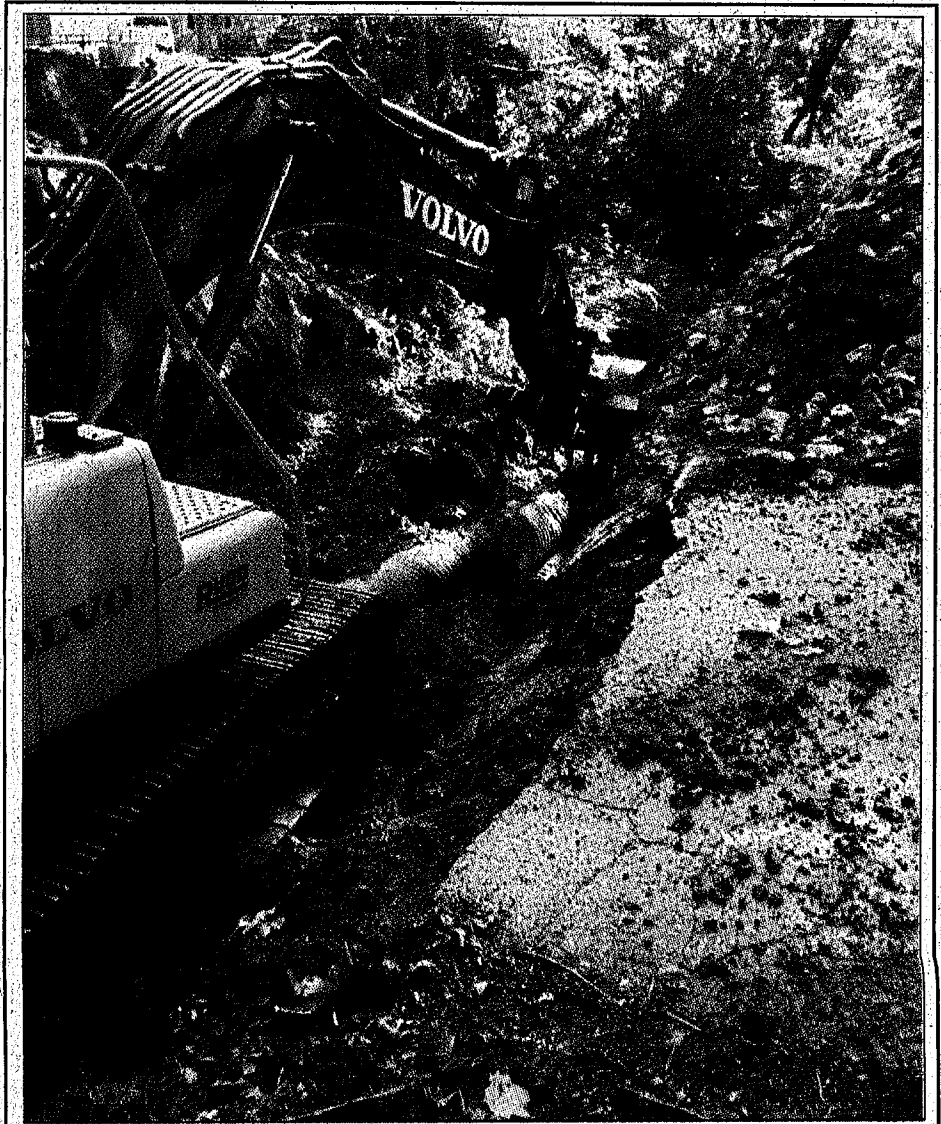
Rockcastle County workers were busy last week replacing deteriorated culverts on Mullins Station Road. The project will cost the county $7,000 and they receive no state reimbursement for the project. The culverts were last replaced in 1993.
