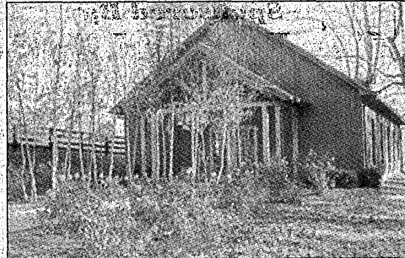
New Construction at Quail Community Park (and no debt)
