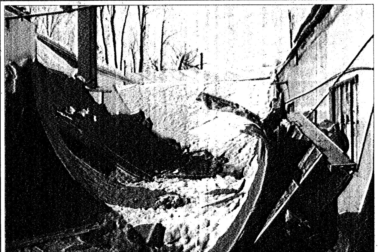
A large amount of damage occurred last Saturday at the former Appliance Service Center building on Hwy 25 in Mt. Vernon. Owners Dale and Laverne Winstead said a large section of the roof in the shop area collapsed due to the heavy weight of the snow. Shown at right is the Winstead's grandson, Conner, standing next to his late father Jeff Winstead's "Memorial Wall" of newspaper clippings of Dale Earnhardt Jr. and other NASCAR memorabilia. The Memorial Wall, located in the shop area of the building where Winstead used to work, survived the roof collapse.
