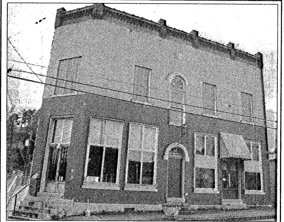
The old Depot Building on Main Street in Livingston was built around 1910 and was left unused since the 1980s until Mayor Jason Medley and many volunteers worked to turn the structure into a community center. The historic building still has marks on the window ledges where men used to stand and sharpen their knives. A gospel singing is held there now each Friday night at 7 p.m.
