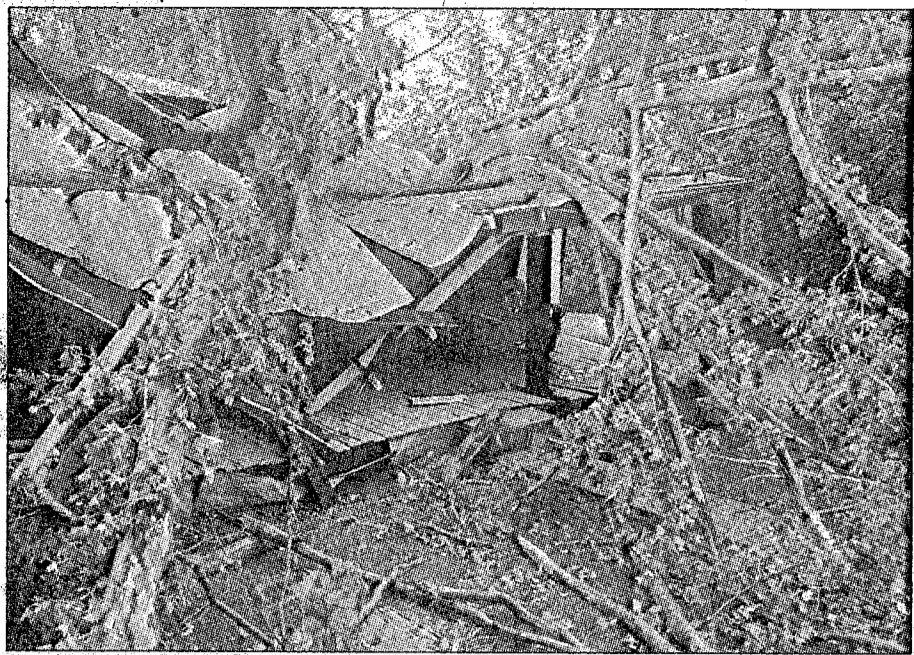
Storms swept through Rockcastle County Saturday night causing damage to some local residences and felled many trees, according to officials. This home on Sweet Water Road was partially destroyed when a tree fell on one side of the home. Though owners were home at the time, there were no injuries reported.
