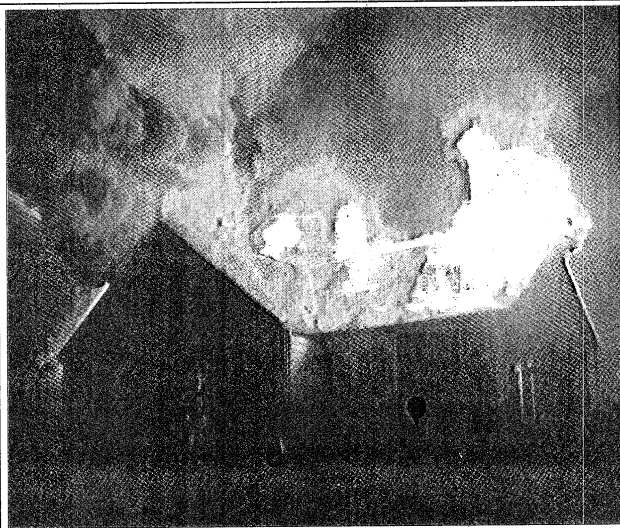
Mount Vernon Fire Department, along with Brodhead Fire Department as automatic aid, was called to a residential structure fire at the intersection of West Main and Williams St. in Mount Vernon early last Thursday morning. This is the same location that saw a fire last Tuesday. Livingston Fire Department also responded for a mutual aid request. The cause of the fire is suspicious in nature and is being investigated by the Mount Vernon Police Department and the Kentucky State Police. If you have any information that may be helpful to this investigation, please contact the MVPD.
